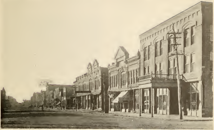
Meridian Street looking South, Portland, Indiana.
